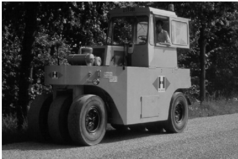
Figure 1.8 A Pneumatic Tired Roller compacting an asphalt road mat (VBW, 2000).
